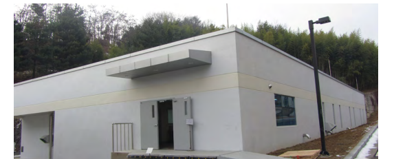
Chemical Storage Facility at Research Park
